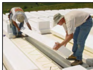
Foam glue is used to attach top-hats to the base section.
