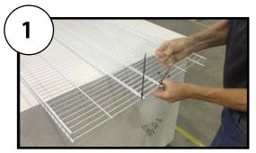
Overlap the Grate so that 1 edge is up and 1 edge is down.
